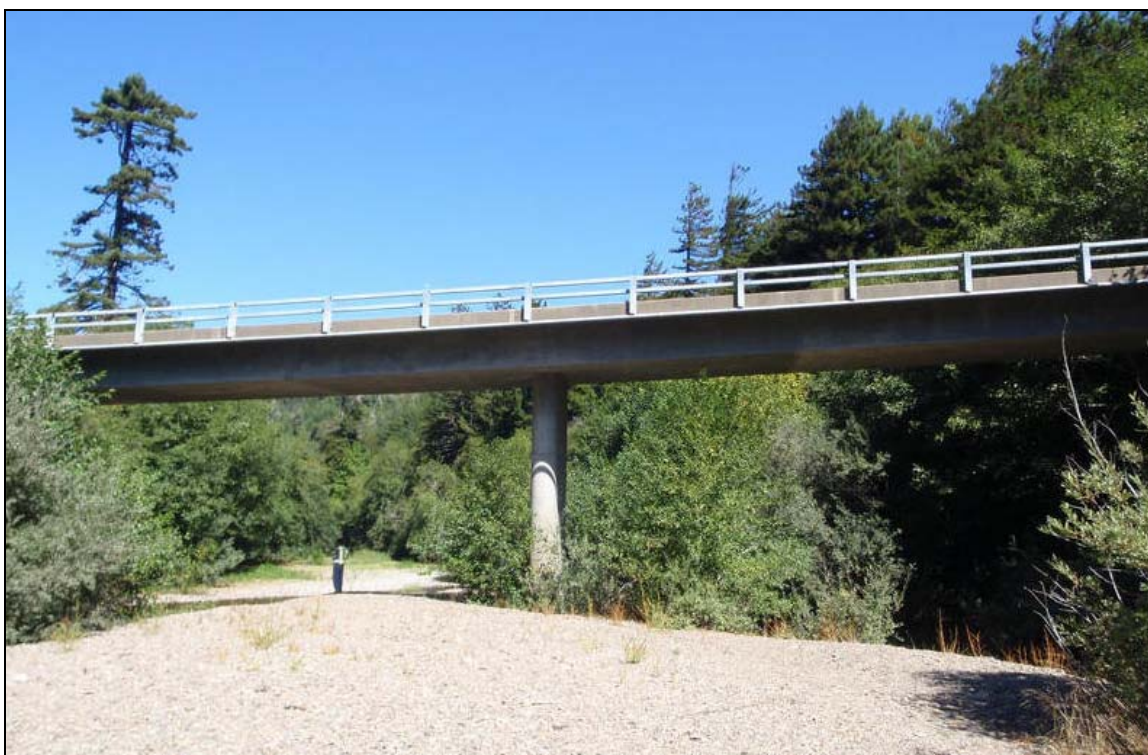
Photo 1. Upstream Face of Bridge (Facing North)
