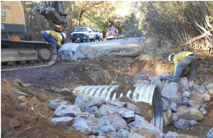
Mendocino County Department of Transportation crew working on a culvert replacement project on Eel River Road.
