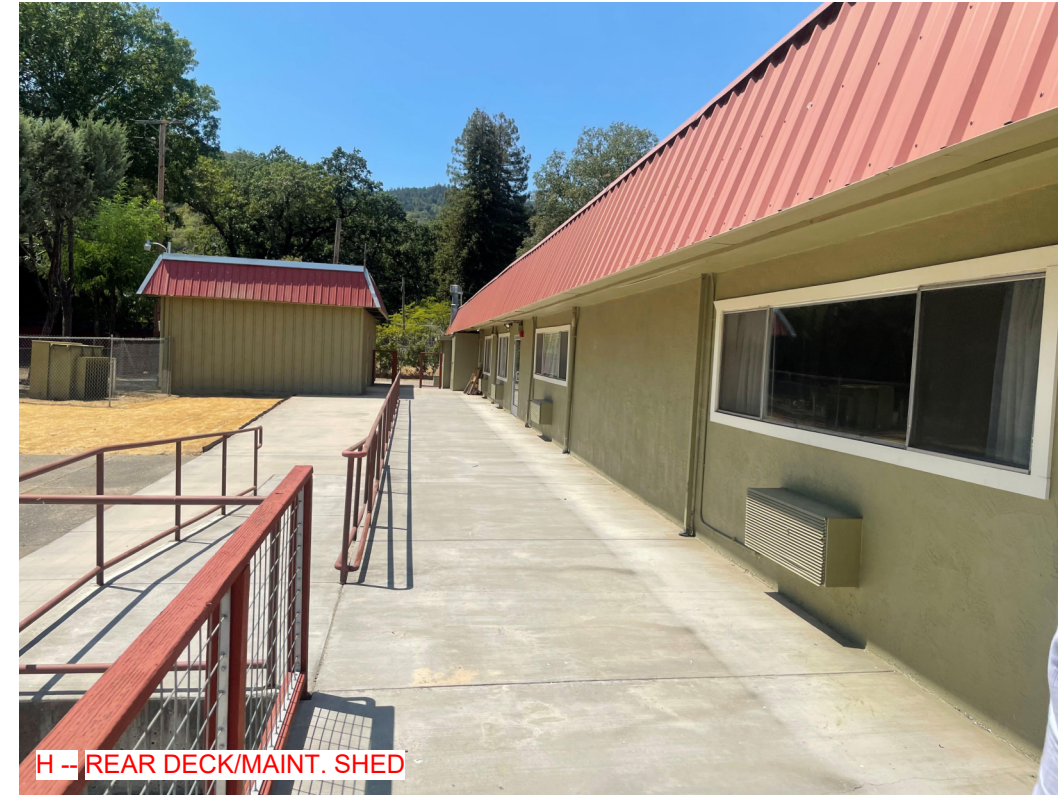
H --REAR DECK/MAINT. SHED
