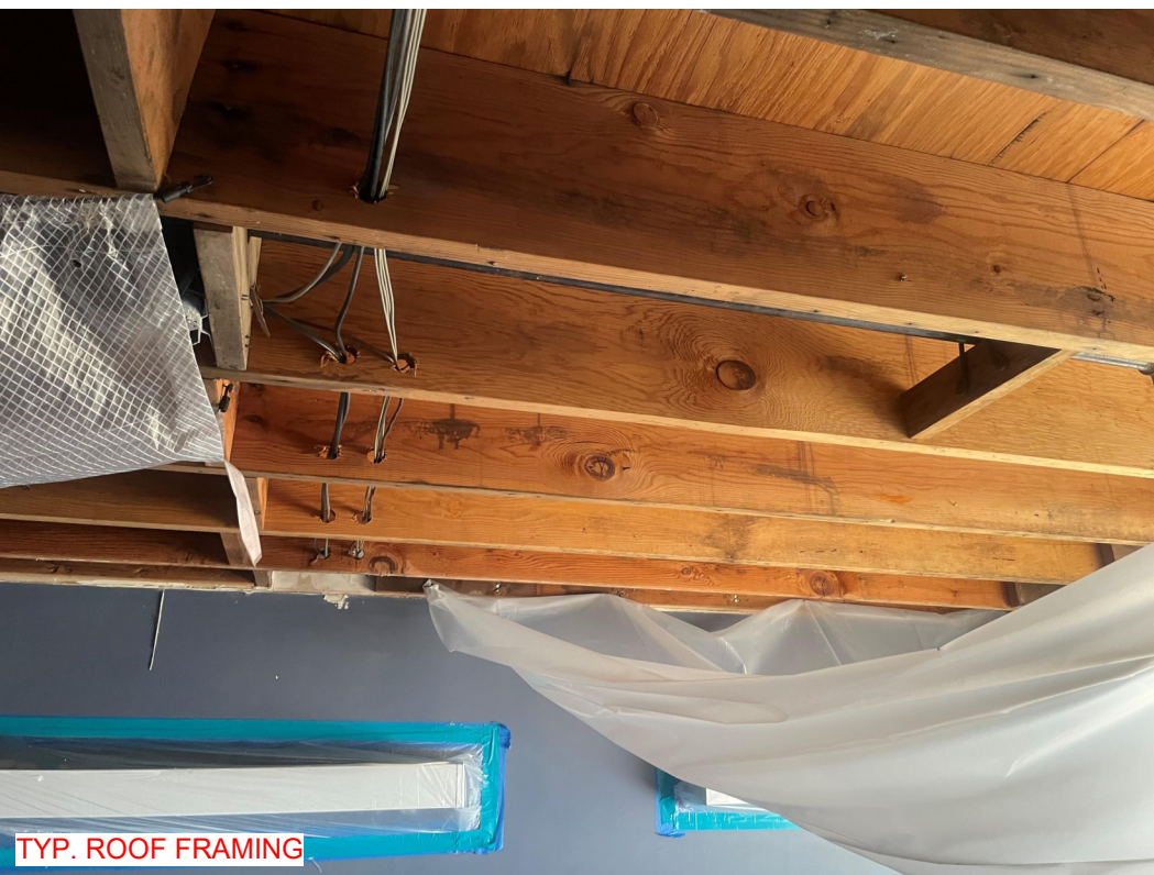
TYP. ROOF FRAMING
