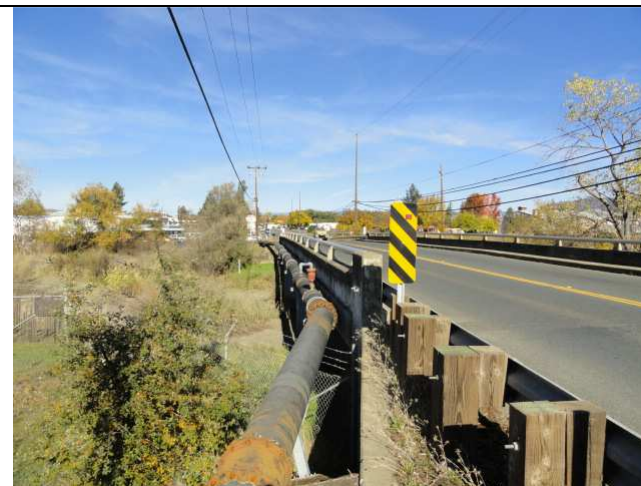
Photo 6: View of water line attached to the west side of the existing bridge.
