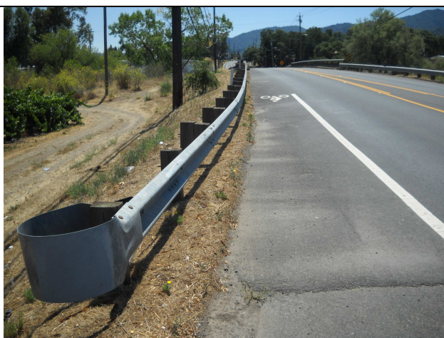
Photo 14: View looking south along east shoulder.
