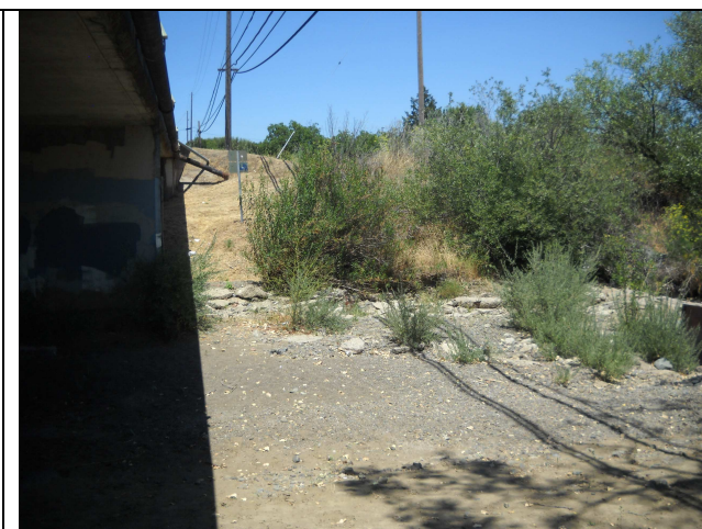
Photo 9: View looking north along the east side of the existing bridge.
