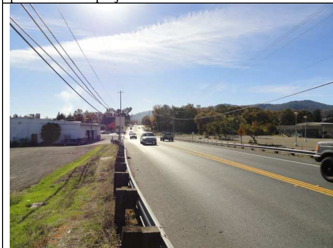
Photo 4: View looking south from bridge along east shoulder of North State Street.
