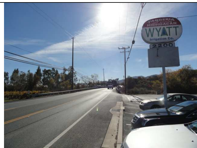
Photo 18: View looking south along west right-of-way toward bridge.
