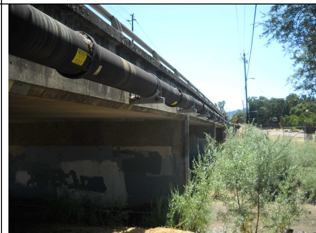
Photo 12: View looking south along the west side of the existing bridge.
