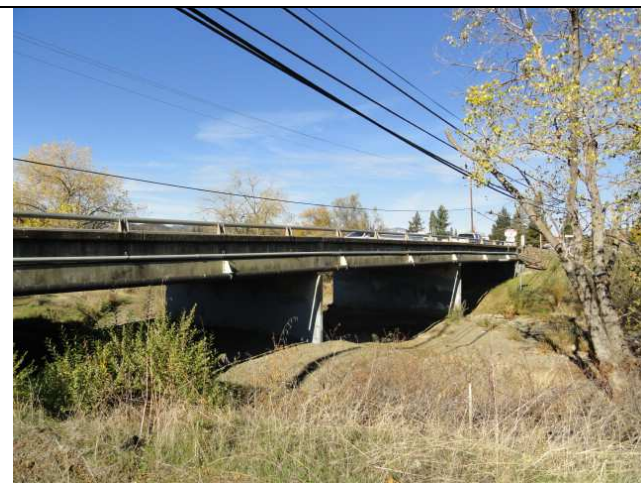
Photo 3: View of the east side of the existing North State Street Bridge.
