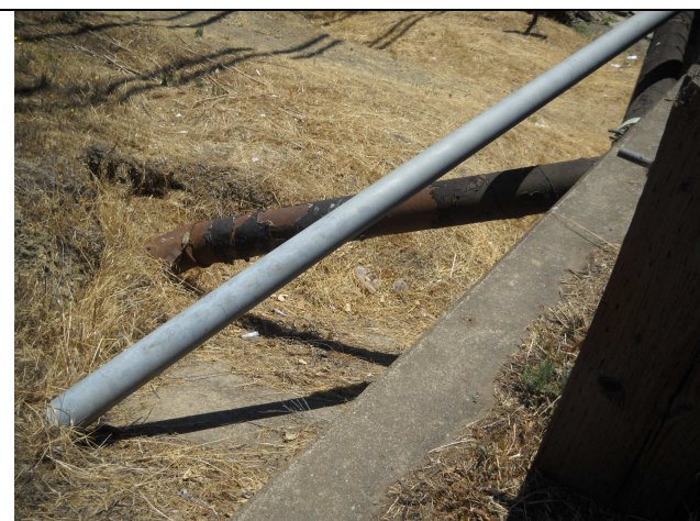
Photo 15: View at northeast bridge abutment showing utility piping coming from bridge.
