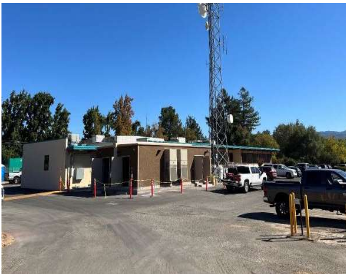
CDBG funded 911 Bunker Building in place
