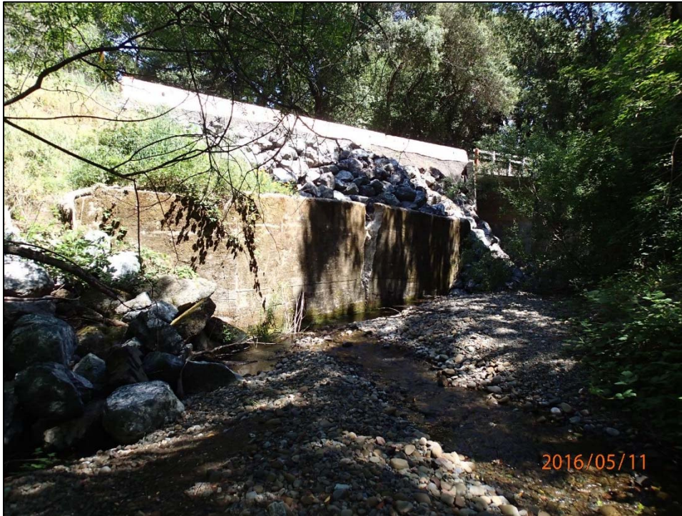
Photo 5. Existing Retaining Wall of Bridge Upstream (May 11, 2016)
