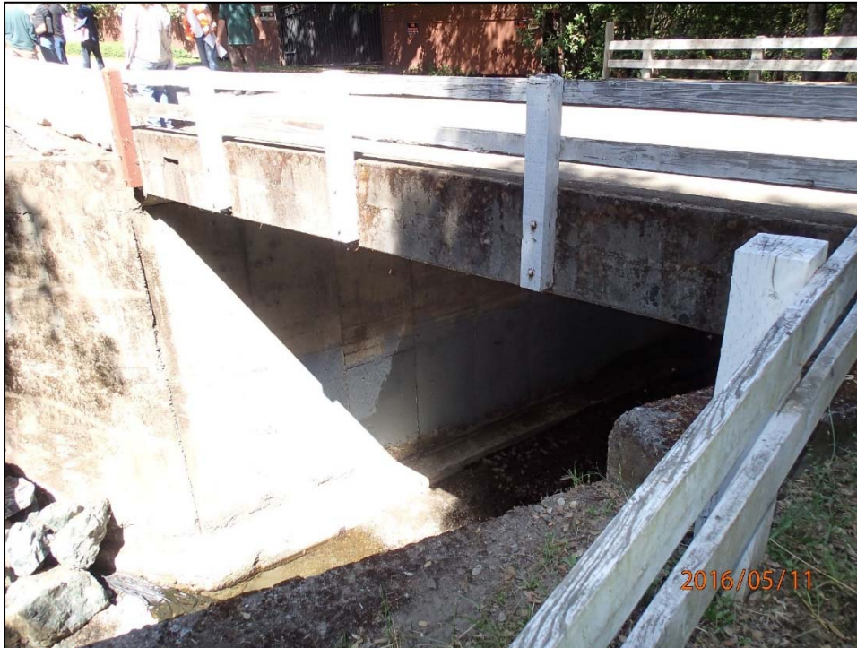
Photo 1. Existing Bridge Upstream Face (May 11, 2016)
