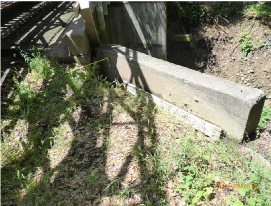
Photo 9. Abutment 2 Offset Wingwall, Downstream Side (May 20, 2019)
