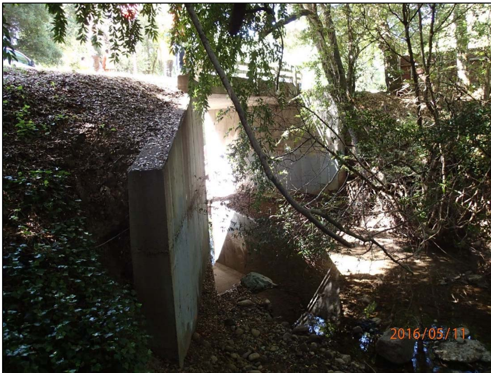
Photo 2. Existing Bridge Downstream Face (May 11, 2016)
