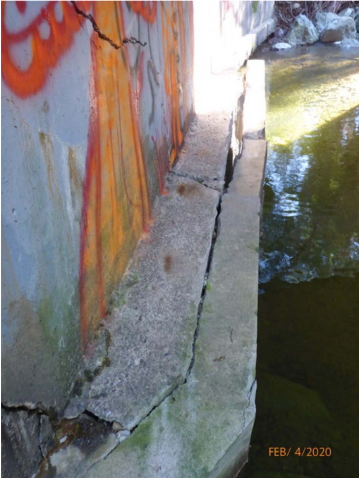
Photo 10. Abutment 2 Foundation, Facing Upstream (Feb 4, 2020)
