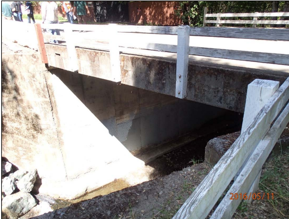
Photo 1. Existing Bridge Upstream Face (May 11, 2016)
