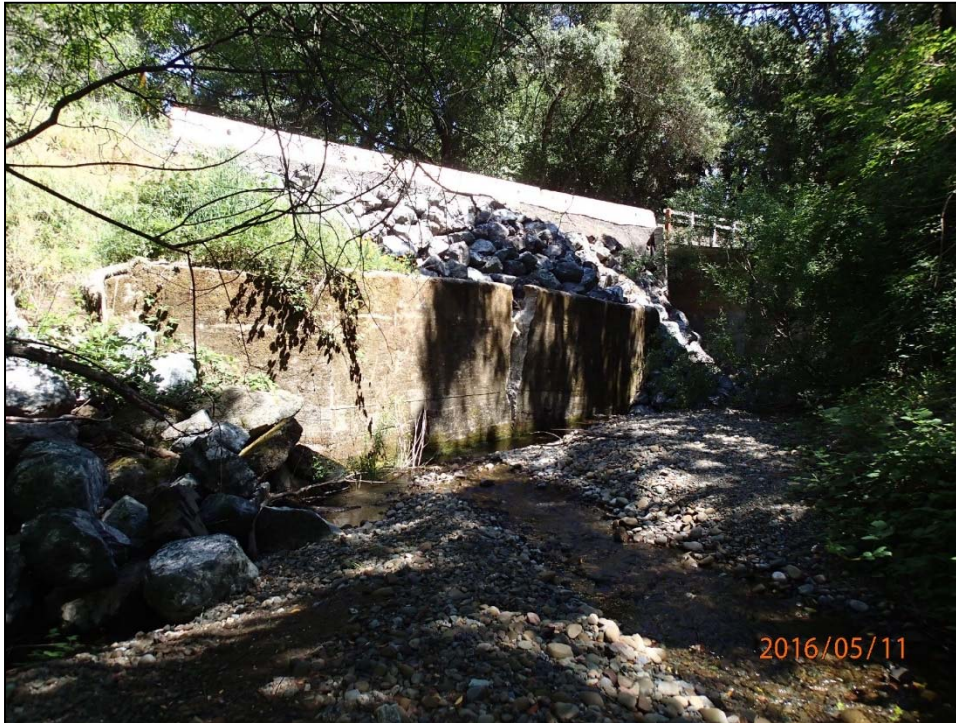
Photo 5. Existing Retaining Wall of Bridge Upstream (South) (May 11, 2016)
