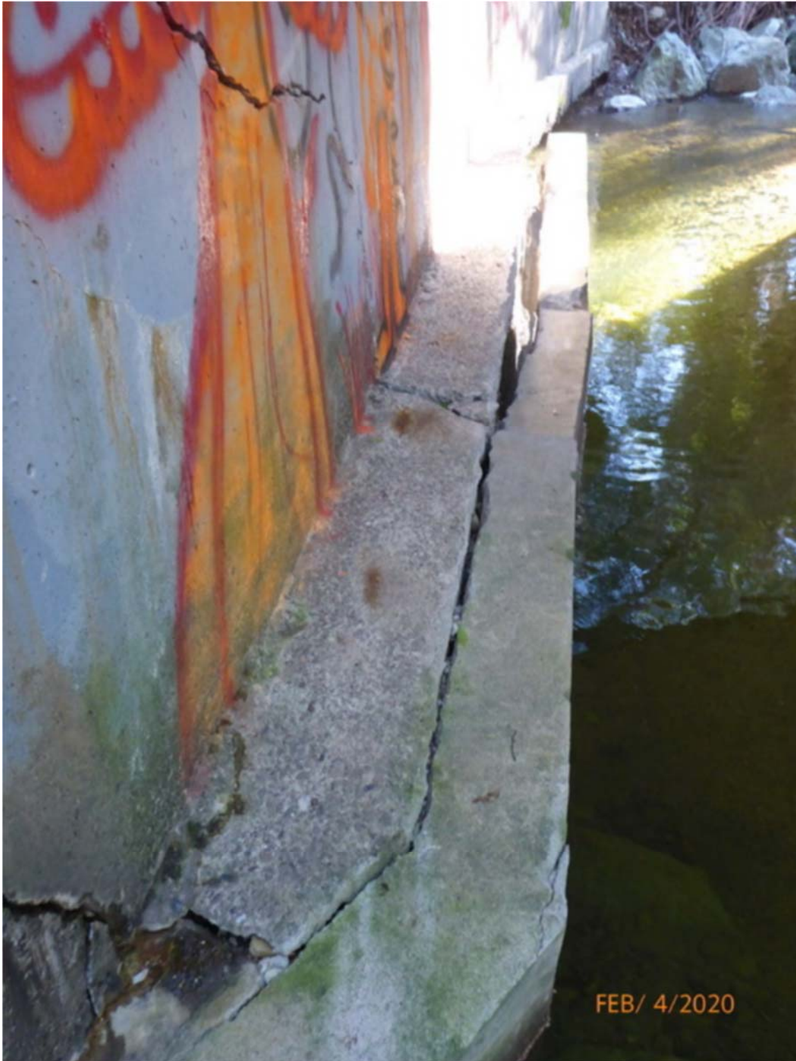
Photo 10. Abutment 2 Foundation, Facing Upstream (Feb 4, 2020)
