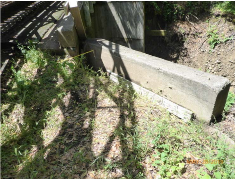
Photo 9. Abutment 2 Offset Wingwall, Downstream Side (May 20, 2019)
