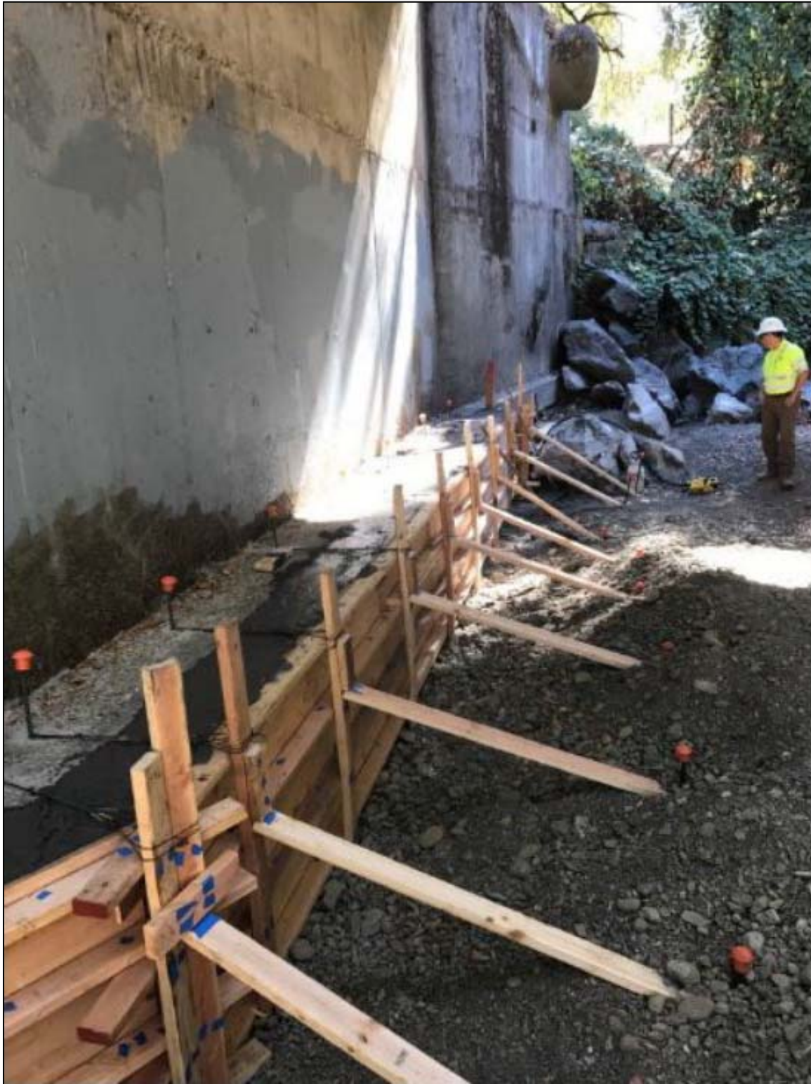
Photo 7. Scour Repair at Abutment 2 (Eastern Abutment) (September 27, 2017)
