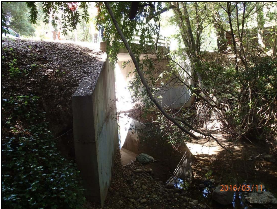
Photo 2. Existing Bridge Downstream Face (May 11, 2016)
