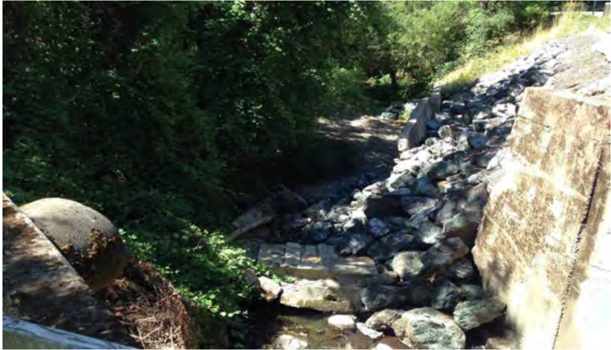
Standing on the northwest corner of the bridge looking west at the failed retaining wall and RSP.
