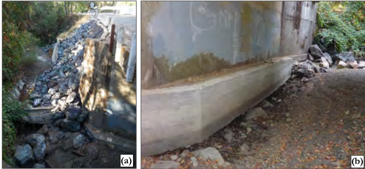
Figure 2. Current condition of the channel at the Lambert Lane Bridge, with (a) riprap placed along roadway embankment at location of collapsed retaining wall and (b) a new concrete skirt along the undermined footing.
