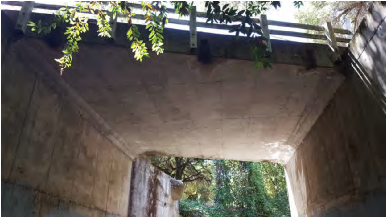
Looking at the underside of the Lambert Lane bridge. No day roosting bat habitat is present.
