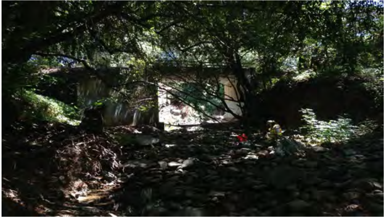
Standing downstream of the bridge looking southeast at the dry creek.
