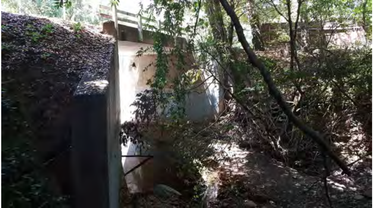
Standing at the southwest corner of the bridge looking north.
