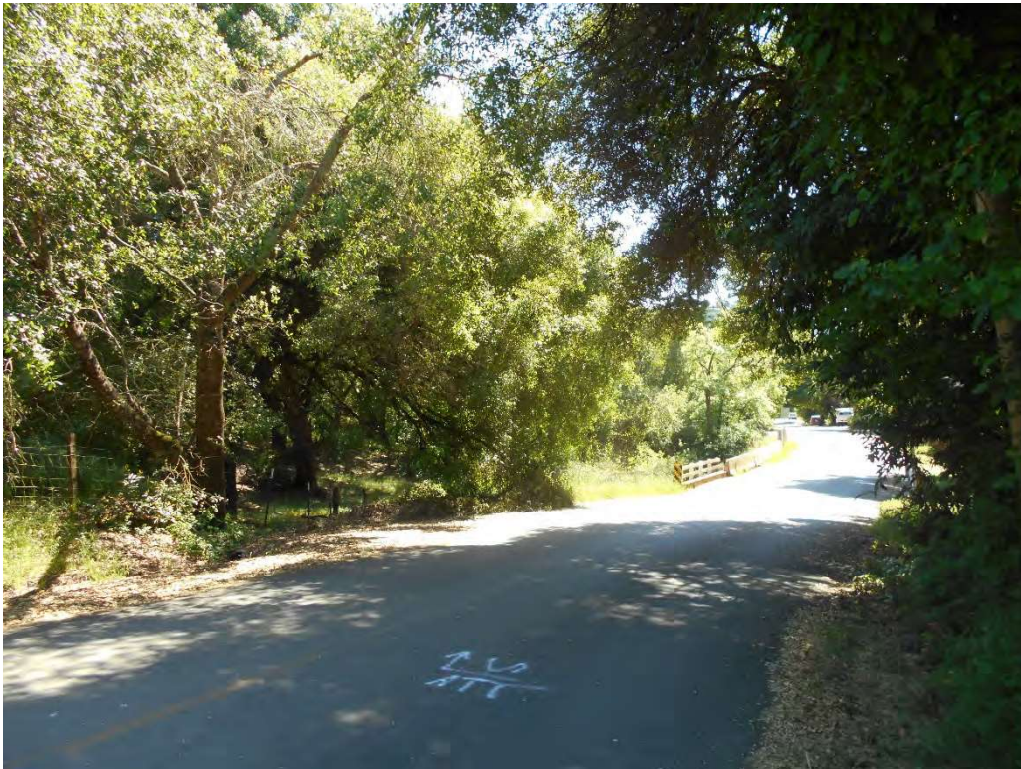
DSCN0610, View southwest, 05/14/2018, Overview of bridge and project area
