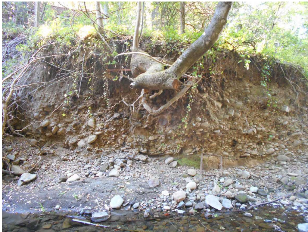
DSCN0614, View west, 05/14/2018, Overview of cut bank on northwest side of bridge
