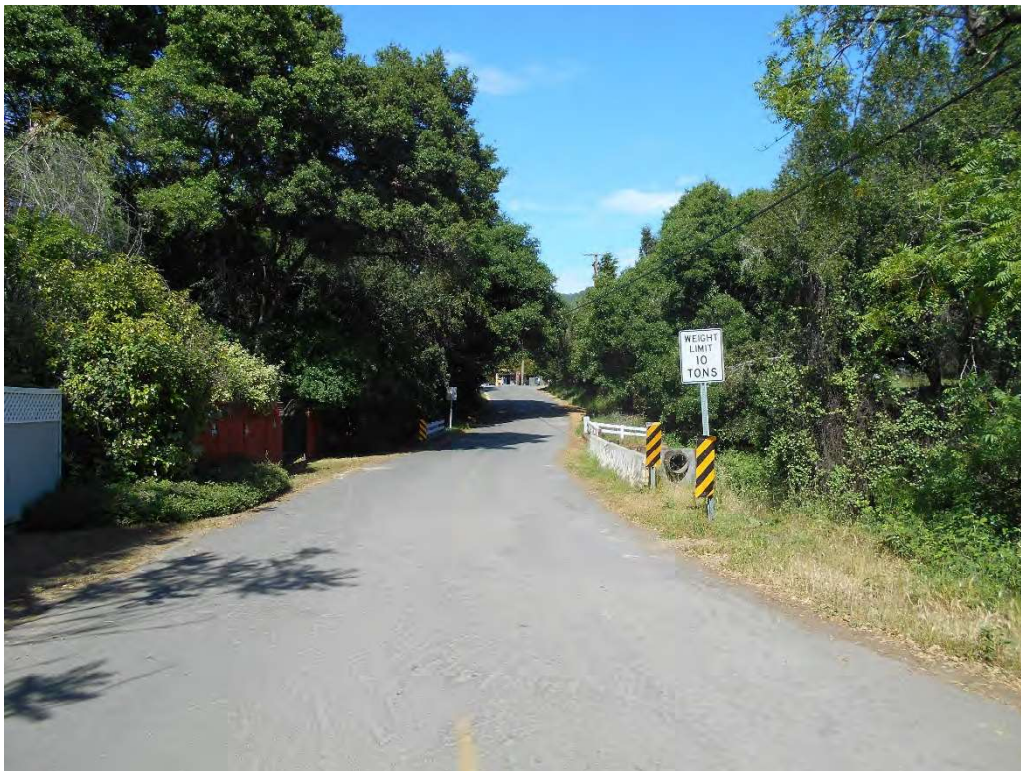
DSCN0618, View northeast, 05/14/2018, Overview of bridge and project area
