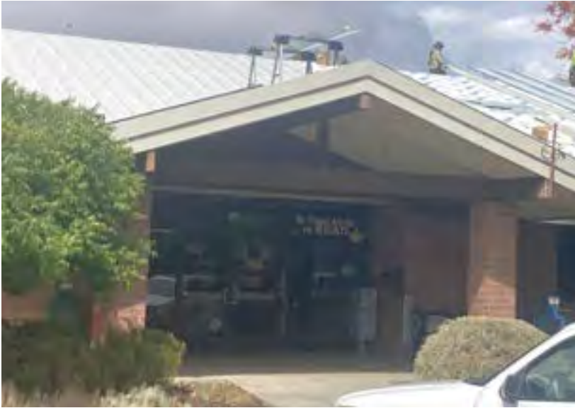
Willits roof construction.
