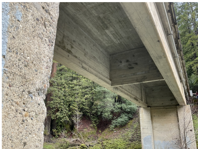
Photo 3 Underside view of Span 2 taken from the right side of Pier 2.
