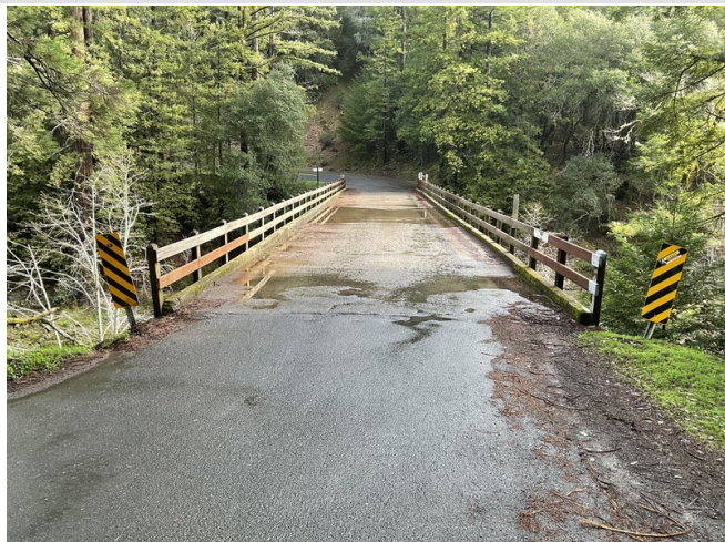
Photo 1 Roadway view taken from Abutment 1.
