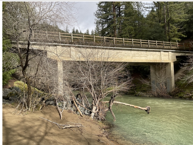
Photo 2 Elevation view taken from the right side of the bridge.
