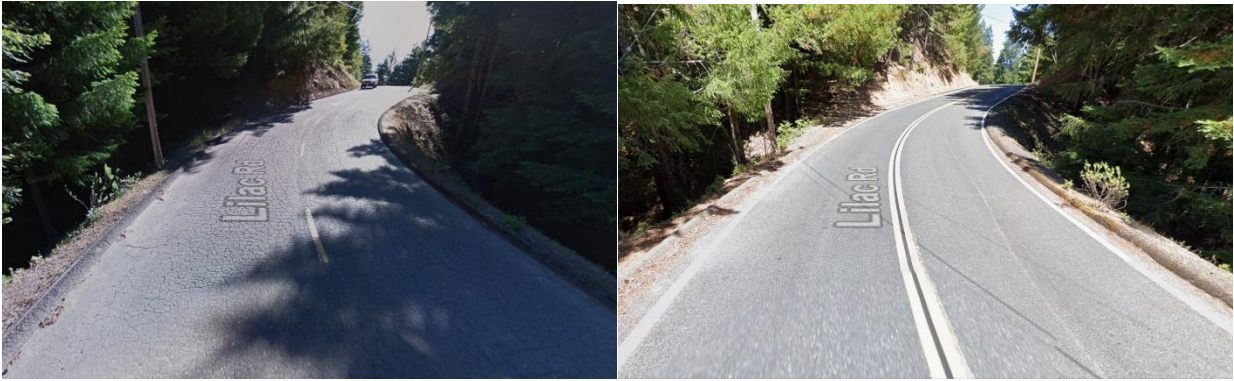
Figure 1. Pictures showing condition on Lilac Rd before (left) and after (right) placing a leveling course and a Double Chip Seal
